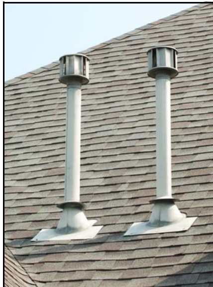
Example of Roof Penetration Flashing
