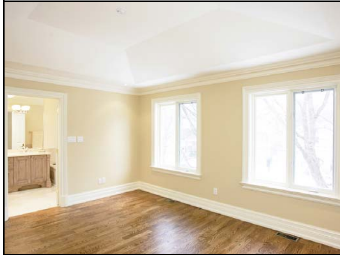
Painted Walls and Molding
