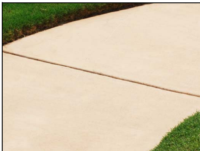
Expansion Joint in Concrete Walkway
