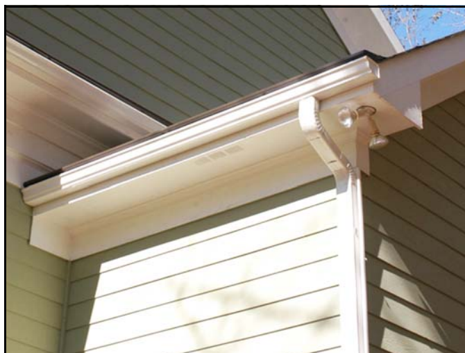
Gutter and Downspout
