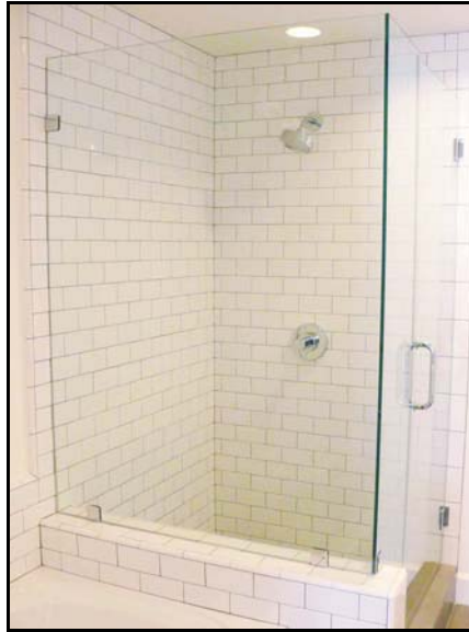
Tile Surround and Glass Shower Door
