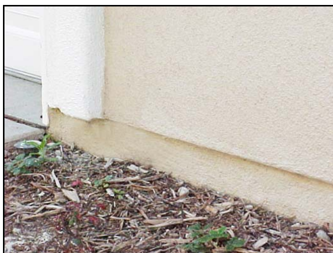
Base of Exterior Wall Finish
